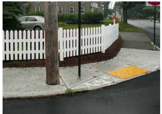
Curb ramp and detectable warning strip
